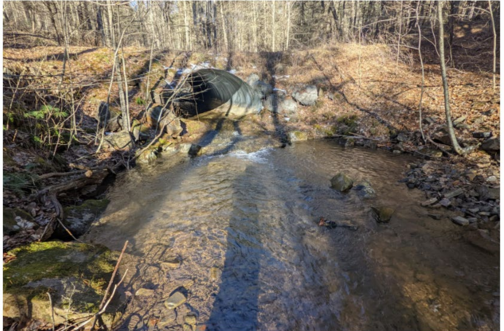
A perched culvert on Virginia's Railroad Hollow creek created a pool that trapped 45 brook trout. TU's Virginia team recently replaced the culvert to reconnect the upper and lower stream sections.
