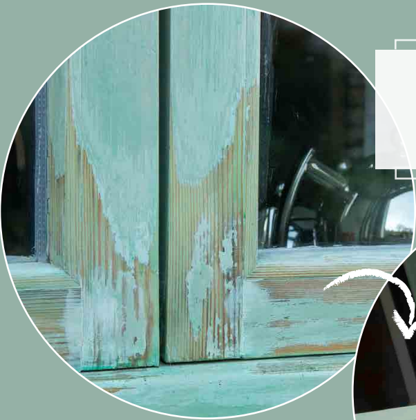
Rotten timber windows in need of some serious repair and maintenance
