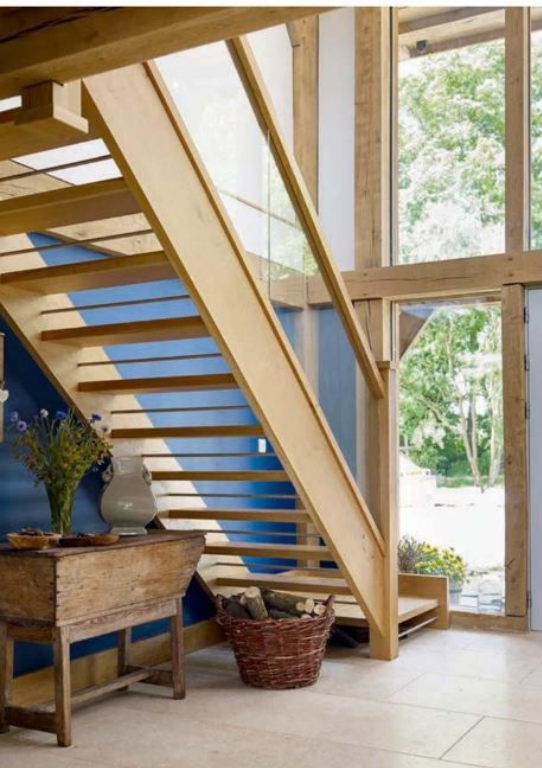
Open treads and a glass balustrade make the staircase design as light and airy as possible
