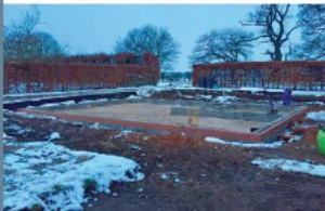
THE GROUNDWORKS AND OVERSITE
