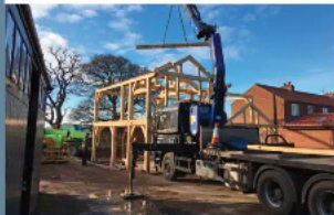
THE OAK FRAME IS ERECTED
