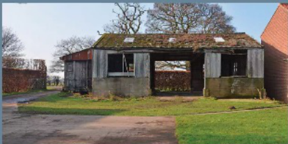
THE ORIGINAL ASBESTOS SHED ON SITE
