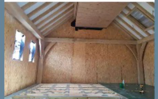
THE FIRST FLOOR INTERIORS TAKE SHAPE
