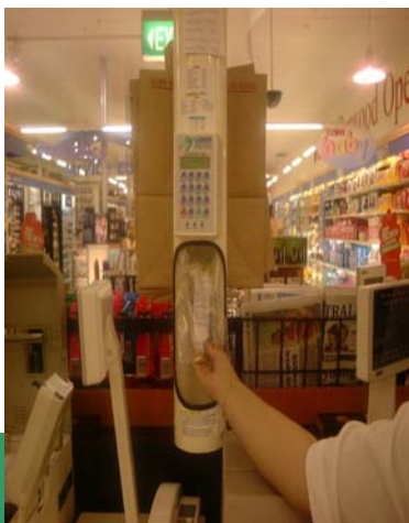
Parachute bag being inserted into a send station
