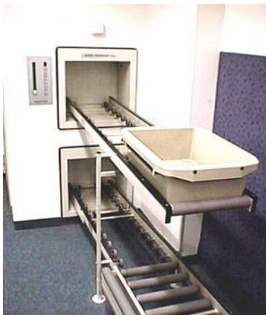
Linear lift container arriving at station
