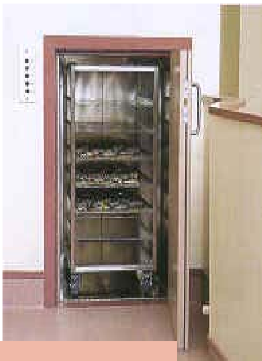
Trolley within lift car
