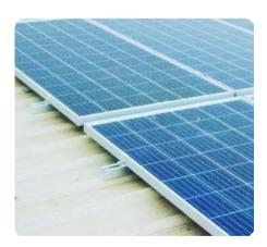
For metallic sheet rooftops, aluminium rail mounting structures work the best
