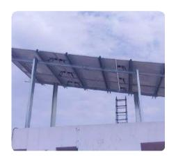
For reinforced concrete rooftops, steel mounting structures coated with a hot-dipped galvanised zinc layer make most sense. The coating makes these structures rust-proof and weather-proof. Most homeowners with reinforced cement concrete roofs prefer taller mounting structures – 6 to 9 ft, to reduce the chance of shadows falling on the solar panels
