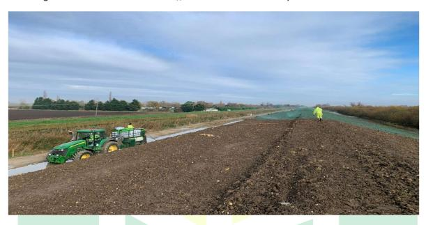
The hydroseeding also needed to provide temporary protection to the slopes whilst ensuring rapid establishment of the grasses and wildflowers.
