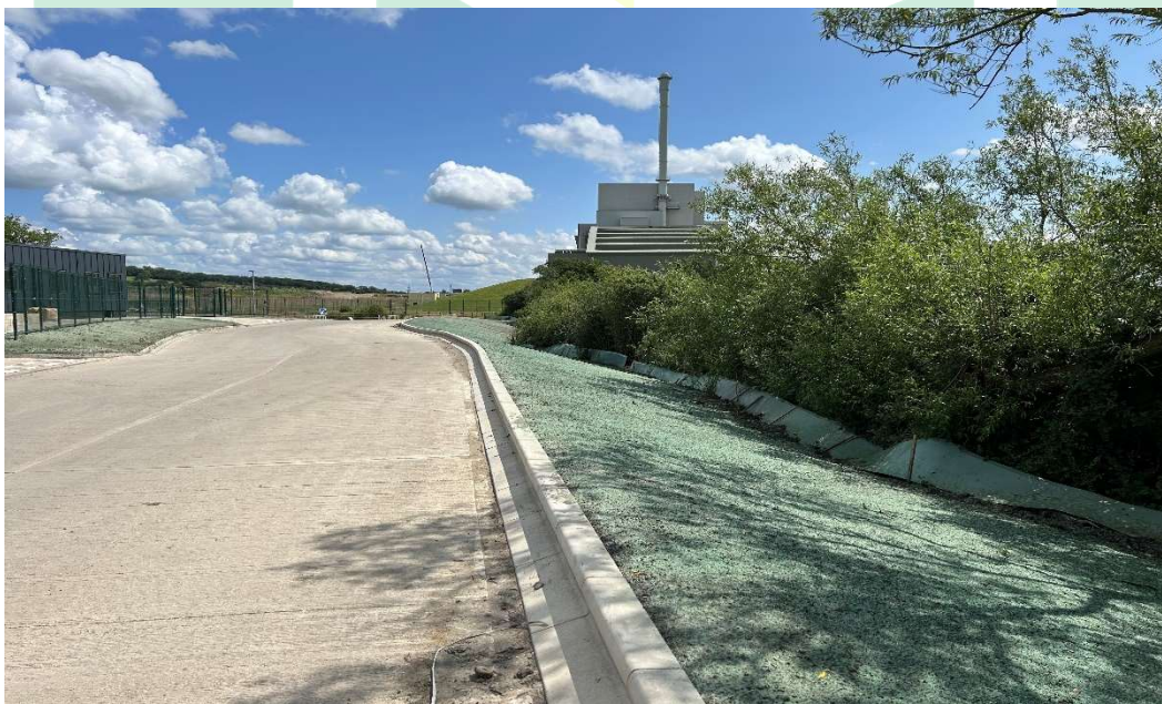
Hydroseeding to verges around of the new landfill site offices behind Greatmoor EFW (June 2023).
