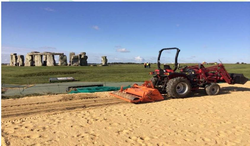
August 2013 - Mixing a thin layer of sand into the topsoil to improve drainage and soil quality using our stone burier as part of the A344 reinstatement work.
