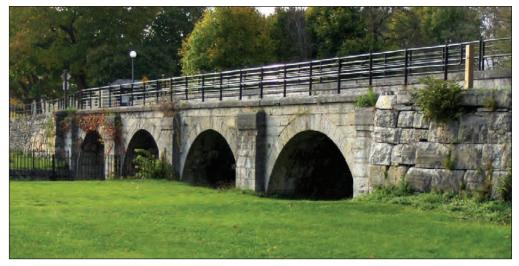
The Jordan Aqueduct was built in 1841 during the canal enlargement. When the bed of the Erie Canal in Jordan was converted to Canal Park during the 1930s, the aqueduct was the centerpiece as a historical record of past transportation methods and development.
