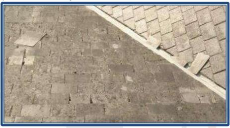
From the line of sight at ground level, the loose slates on this pitched roof could not be seen and had managed to go unnoticed for an unknown length of time.
