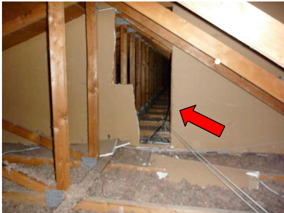
Photo #7: damaged firewall
