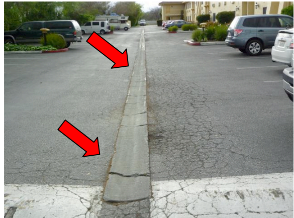
Photo #17: damaged pavement
