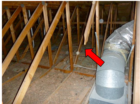
Photo #6: broken truss
