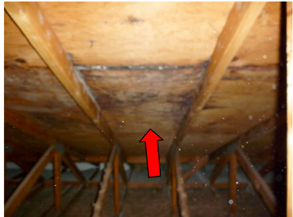
Photo #11: roof leak w/ plywood damage
