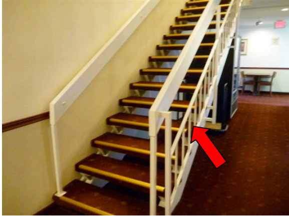
Photo #1: non-grippable, 4" openings
