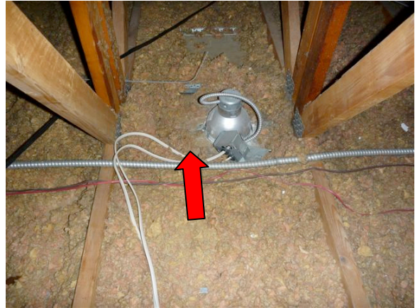
Photo #5: romex wire in attic
