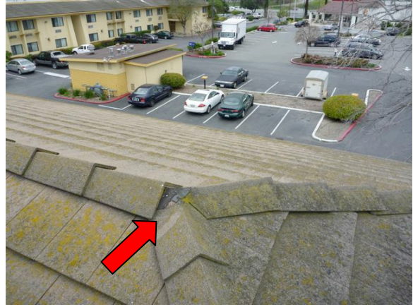
Photo #4: weather cap missing here
