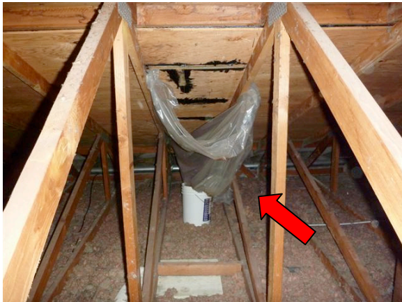
Photo #8: roof leak w/ patches
