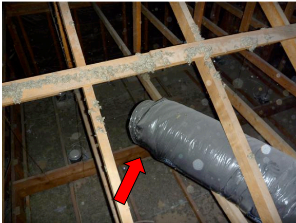
Photo #14: disconnected heating duct
