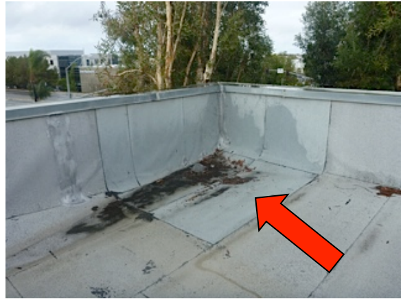
Photo #10: debris at corner drain
