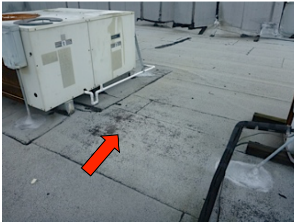
Photo #14: aging roof surface
