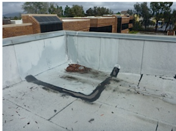
Photo #12: past roof corner repairs
