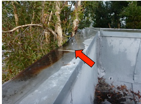
Photo #11: water pools on parapet
