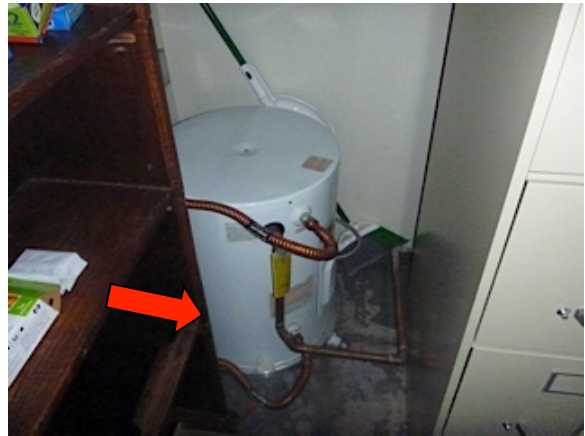
Photo #16: pan drain not to exterior
