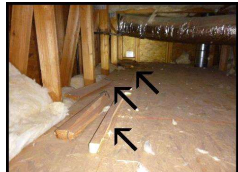
remove wood scrap from attic here
