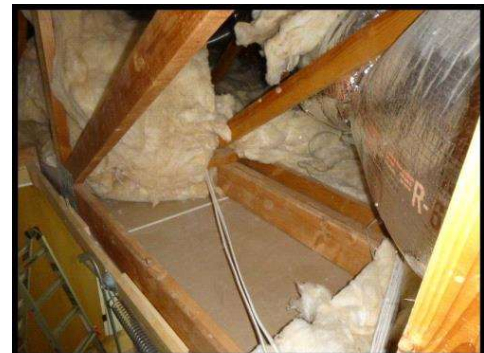
insulation gap example
