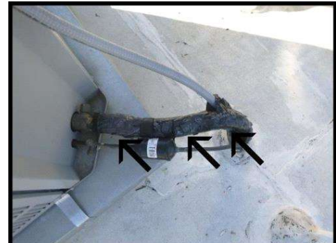
redo insulation with vapor tape
