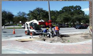
"These machines allow co-op line workers to set new poles or replace downed poles in areas of limited access. They are well-suited for storm restoration be it blizzard, tornado or hurricane, to help line crews work safer and more efficiently."
