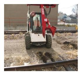
The Rail Tool makes it a snap to insert new crosstie into place.
