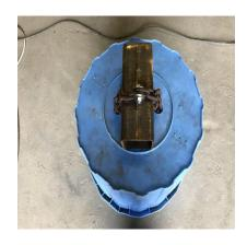
6. Check your anchor placement turn your tub back upside-down, place a 4 X 4 between the hole and Bring your chains up around the 4X4 and secure the two ends of the chain with a nut and bolt.
