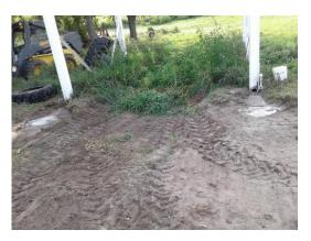
10. Dig holes and bury one concrete block, chain side up, where each leg of your bin will rest on them and your chains will join at the top of the runner.
