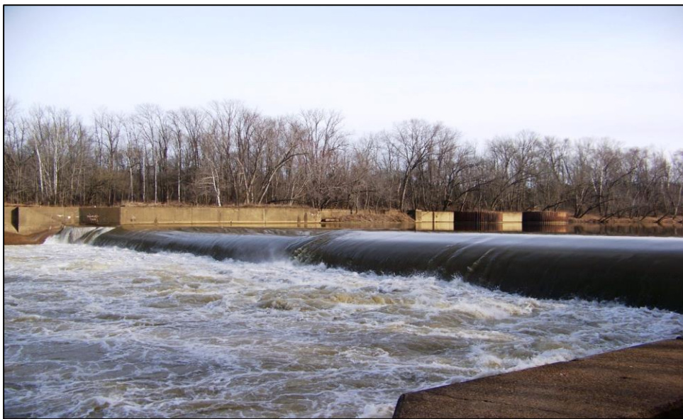
Lock and Dam 5
