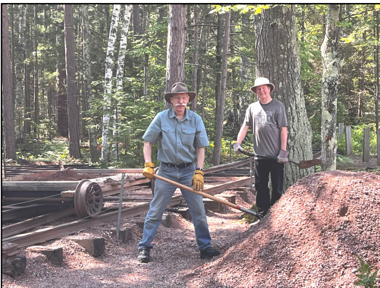
Paul Johnson and Tom Tardiff shoveling gravel as ballast.
