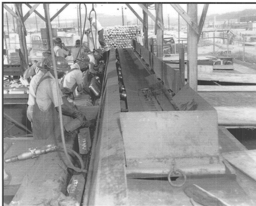
Photograph 4: Workers emptying flasks of mercury at the Y-12 mercury dumping shed. Pipelines carried mercury to the buildings that housed the Colex operations. (1955 photo ORO-55-762-3 courtesy of U.S. Department of Energy)
