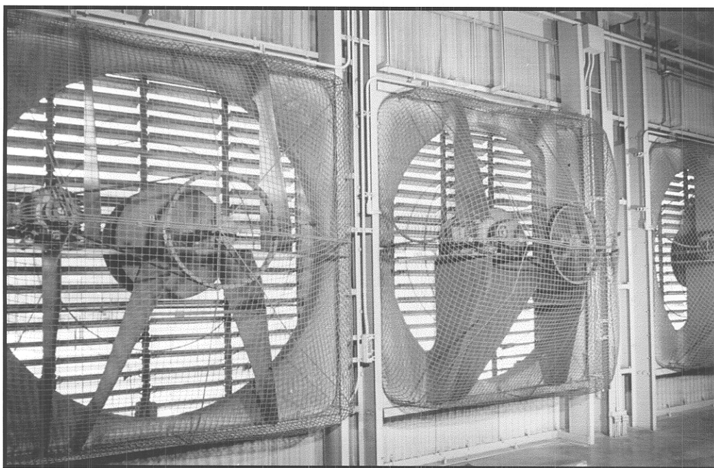
Photograph 5: Six-foot diameter fans were installed in Colex Building 9201-5 in 1956 to increase ventilation and thereby reduce airborne mercury concentrations in operating areas (Photo 102455 courtesy of the Y-12 Plant).
