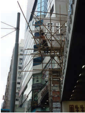
▲ Workers putting up bamboo scaffolding in Hong Kong
