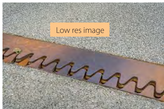
Figure 9.6 Expansion gaps in a bridge roadway
