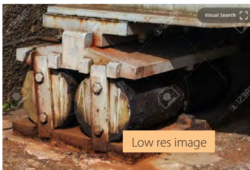
Figure 9.7 Rollers supporting one end of a bridge
