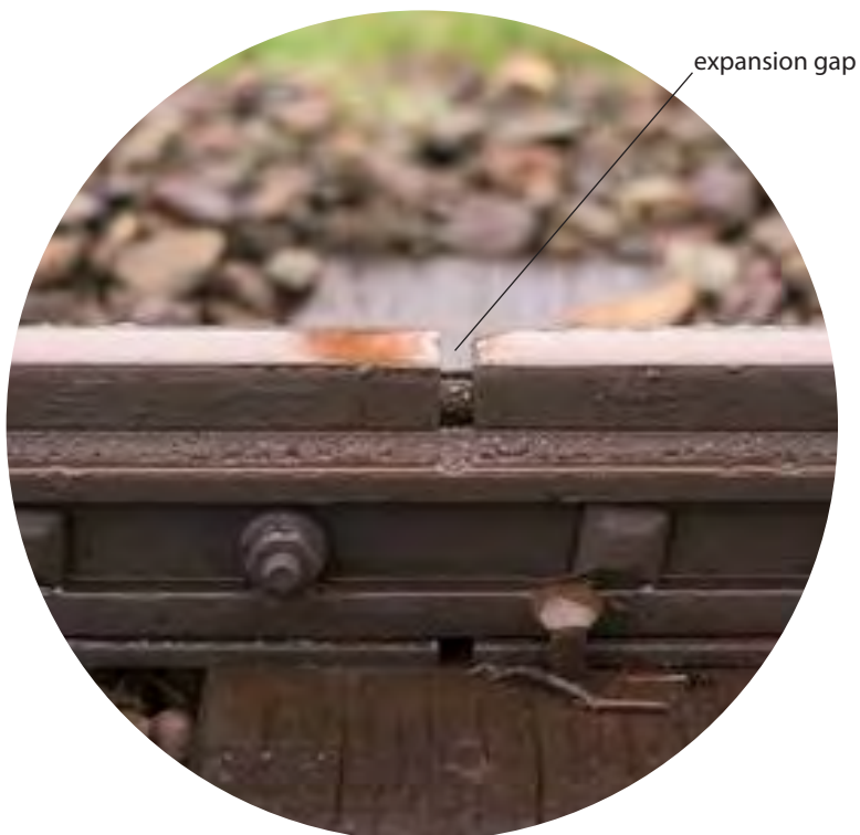
Figure 9.5 Expansion gaps in a length of rail
