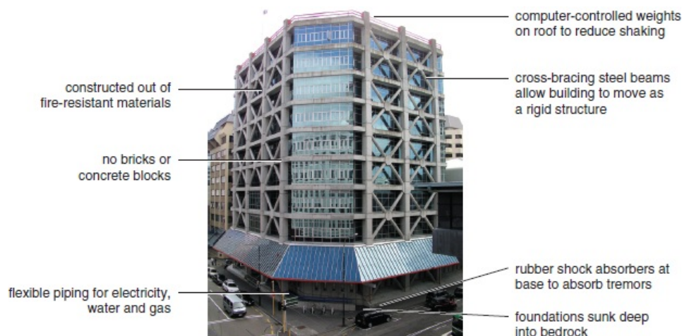
Figure 6.14 Some features of an earthquake-proof building.
