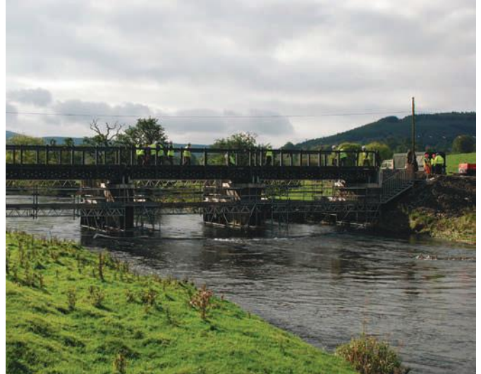
Figure 21.34 The world's longest bridge made from recycled plastic. It was constructed in Peeblesshire in Scotland.
