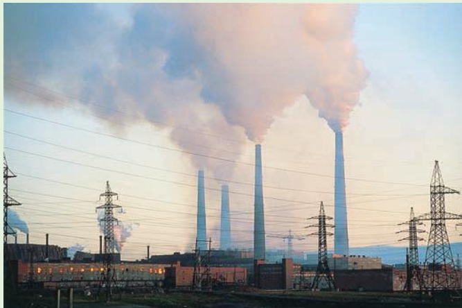
Figure 21.25 Air pollution by industry. Tall chimneys keep pollution away from the immediate surroundings but the atmosphere is still polluted.
