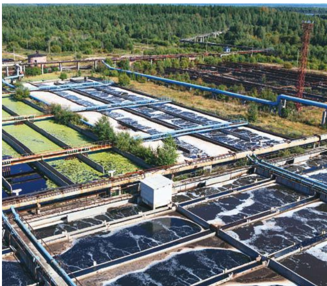
Figure 21.36 Sewage treatment – activated sludge method. In the foreground are the rectangular aeration tanks.
