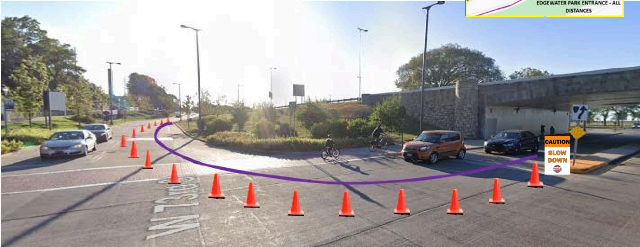
W. 73rd Street to Edgewater Park Entrance
