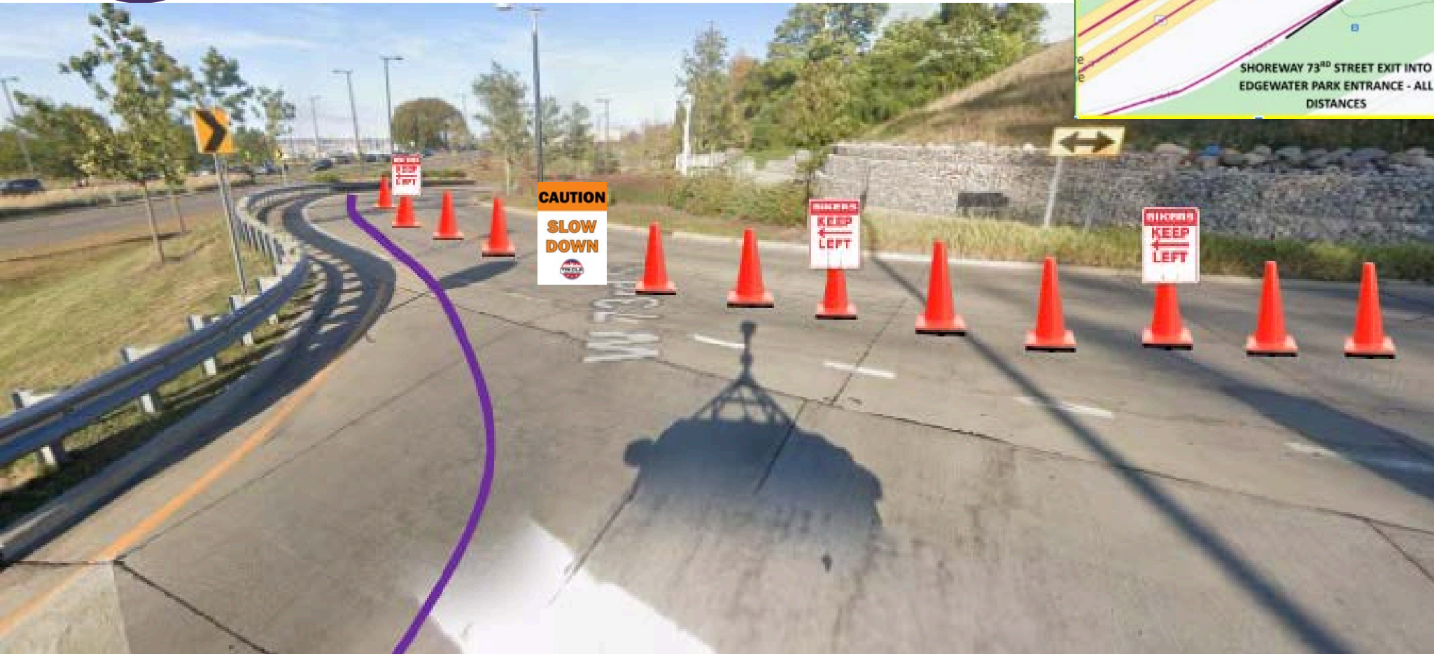
Shoreway Exit to W. 73rd Street
