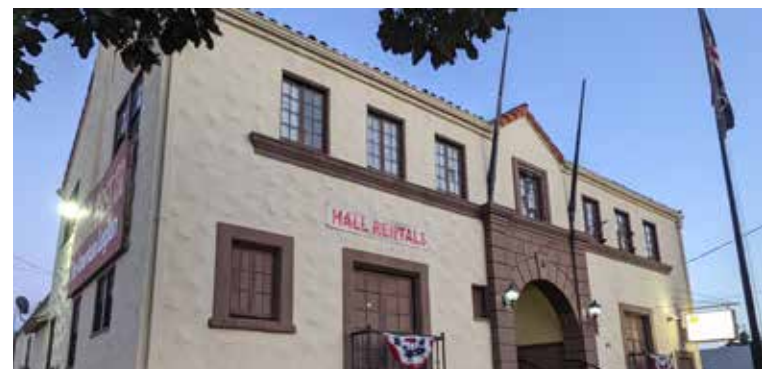
New windows have spruced up the American Legion Post building.
