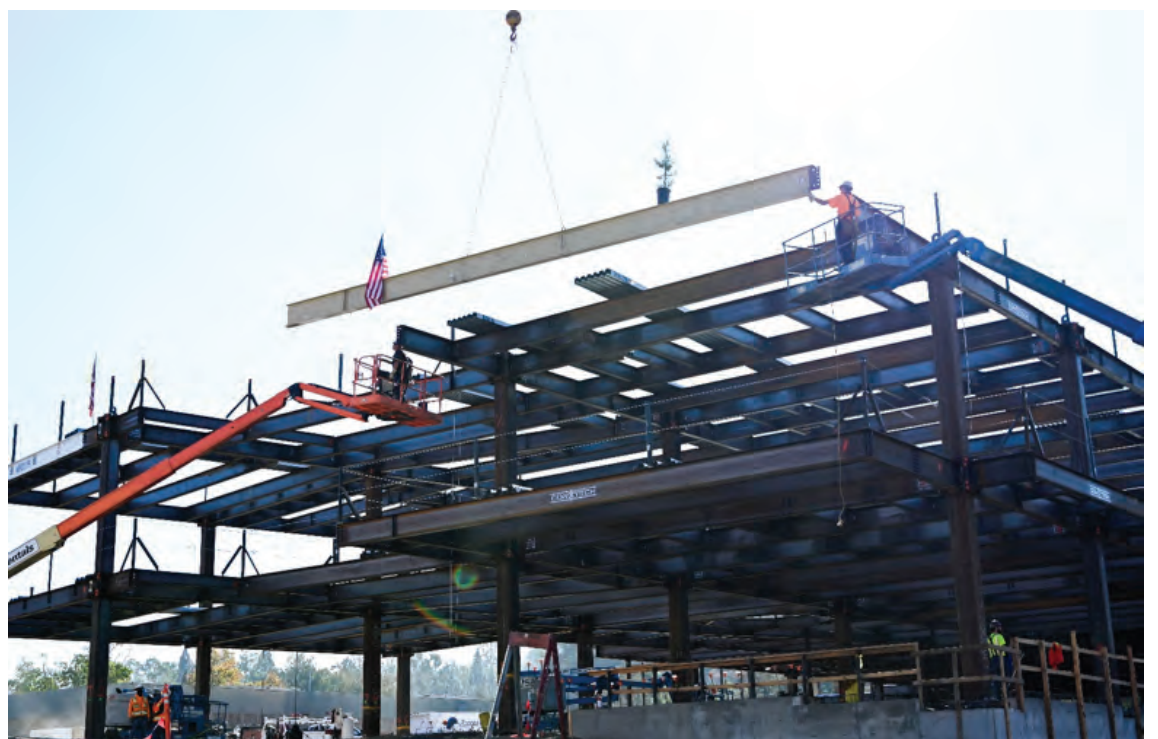
The final steel beam was lifted into place on Canyon High School's new state-of-the-art science center, Nov. 19. Canyon's 67,098-sq.-ft. building is one of four paid for with funds from Measure S to bring Orange Unified high schools into the 21st century. In addition to modern science labs and classrooms, the building will serve as a "front door" to the campus and house student support services. The final beam was signed by students, staff, administrators, community members and elected officials.
