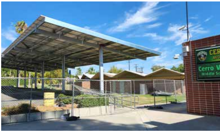
Parking lot shade structures with solar roof panels are being installed at Orange Unified schools (Cerro Villa Middle School, shown here) over the summer. The district estimates that $7.8 million in OUSD electricity costs will be saved over 25 years.
