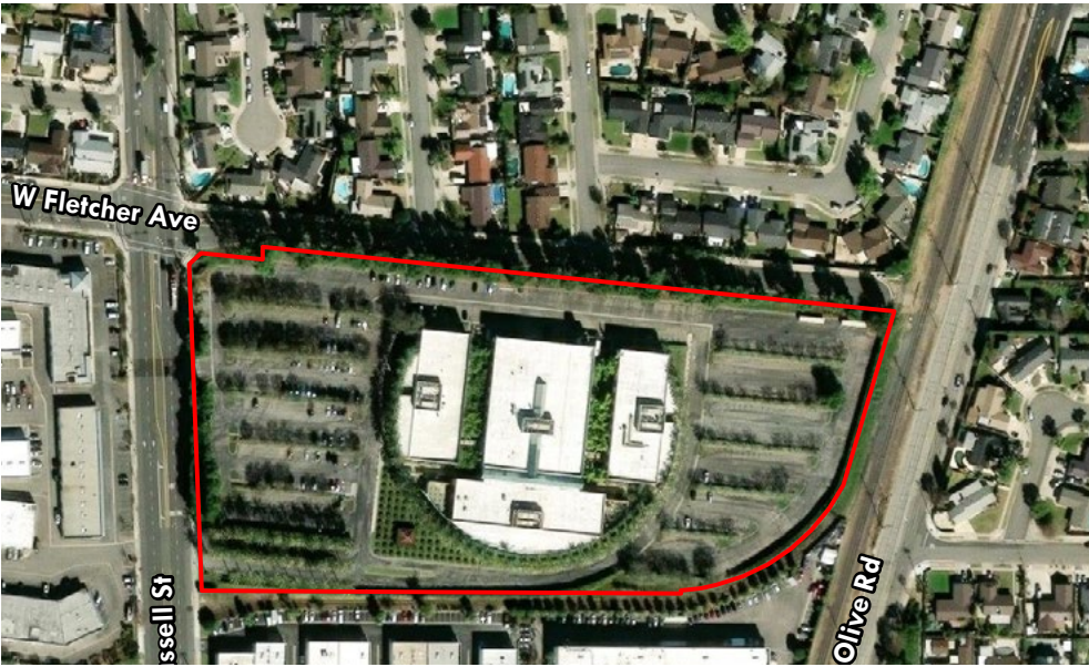
Aerial view of the proposed truck terminal site
