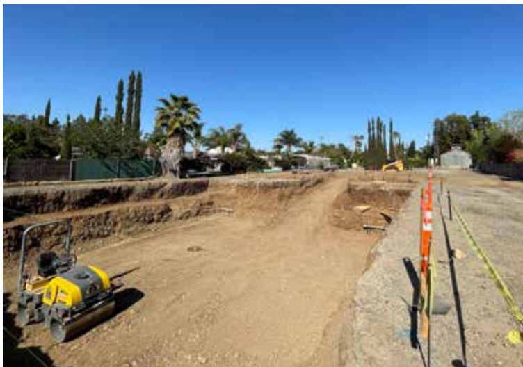
Ground was broken for the OCWD PFAS treatment facility, April 12, to be built on SWD property in Villa Park. The structure, which will rise only 10 feet above ground, is slated for fall completion.
