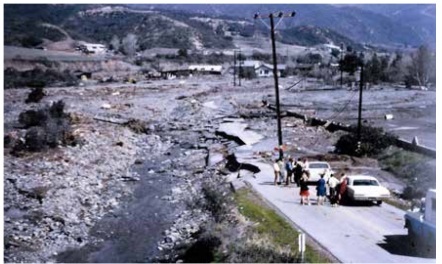
A torrent of Santiago Creek floodwater took out a road in 1969.
