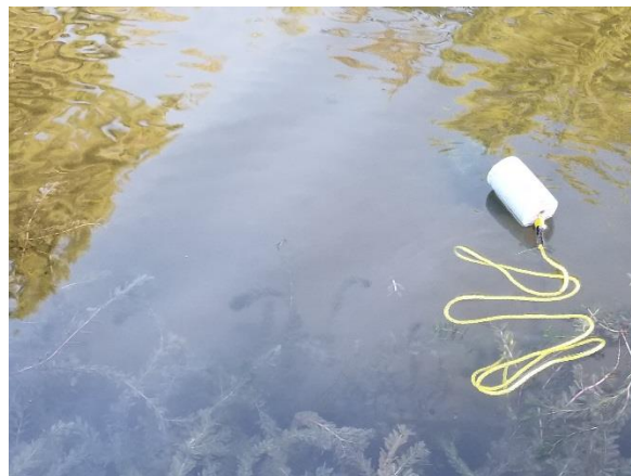
Rope and float to keep track of the rebar for easy pick up
