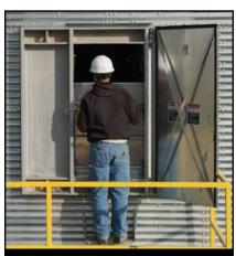
Brock Latch-Lock® Walk-Through Bin Entry Doors offer safe, convenient access with an inner and outer door frame and interlocking inner panels that open, in sequence, from top to bottom, with a lift of a latch.
