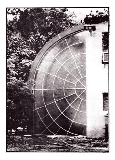
System Description: Greenhouse heated air is cycled down through air ducts located within laminated wooden columns to subfloor thermal mass storage. 6 1/5 HP fans supply the heated air across 2800 recycled one gallon plastic containers filled with water which make up the subfloor heat exchanger. A seperate room fan air loop crosses through the exchanger in a cross flow configuration to supply heat to the building.
