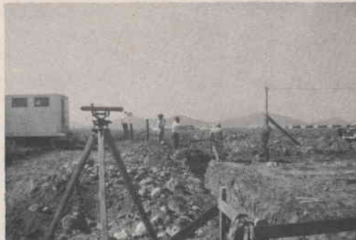
First day of work. Trenches are dug for footings.
