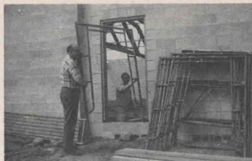
With outside walls up scaffolding is set up.
