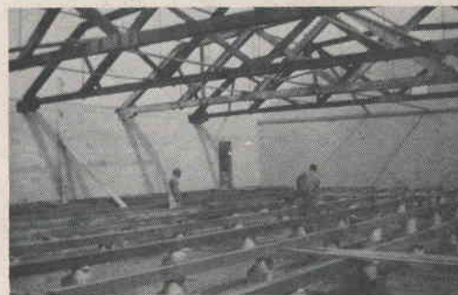
Trusses are set and floor joists tightened.
