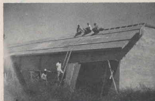
Sheathing is applied prior to the asphalt roofing.
