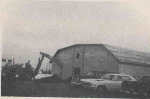
Exterior of building as it nears completion.
