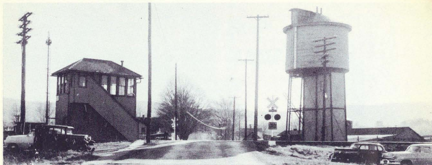
UNION STREET CROSSING shown here is a good place to be on the alert. Poor visibility caused by water and signal towers add to hazard; heed those red flashers.
