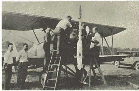
On September 28, 1929, Jimmie Doolittle flew the Guggenheim Fund Plane (a Chance Vought "Corsair"), used in connection with fog flying experiments, to Sidney for installation of a Rome wire harness and radio shield. The above Scintillites made the installation, at the same time checking over two Scintilla VAG9D mags. From l. to r. — Warren Kishbaugh, August Asplund, Al Herdecker, Al Jacobs, Robert Graham and Jerry Walker.
