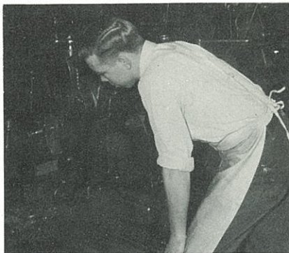
For his first on-the-job training assignment as an apprentice, Benjamin DeMott was instructed in the use of a shaper.
