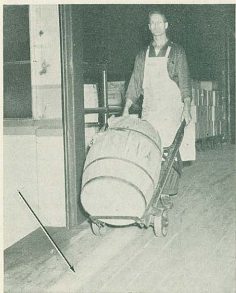
Arrows point to Safety-Walk installed in Shipping and Receiving Dept. ramps. Strip of abrasive material cemented to concrete provides safe, non-slip footing for employees engaged in loading and unloading operations. Coming down Receiving ramp is Don Codgington, while Ray Borden finds the Safety-Walk helpful in pushing loaded truck up Shipping ramp.
