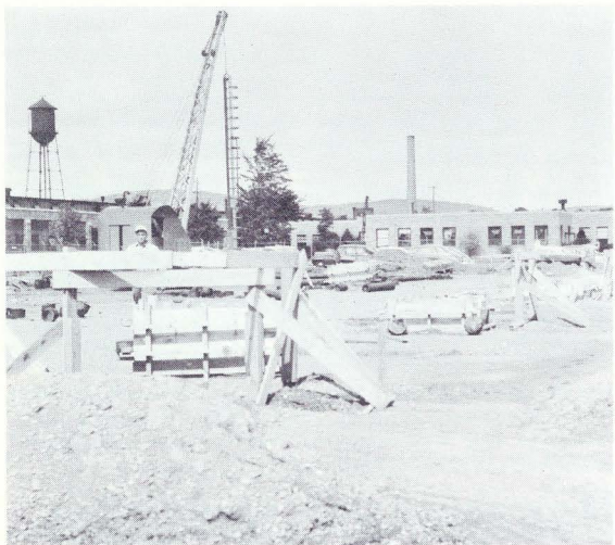
SCINTILLA'S latest expansion of plant facilities is taking place at West end of factory.
