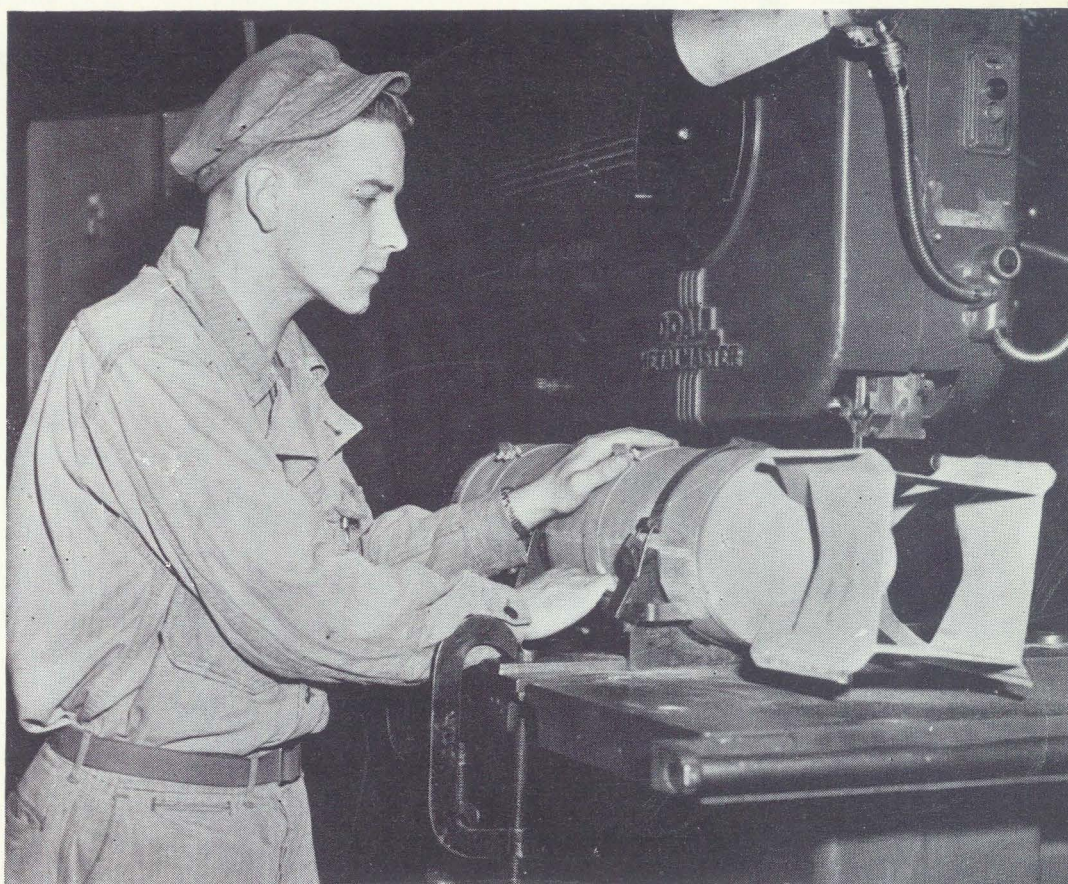
A clamp brace constructed by Cpl. Elbert Bartlett, former apprentice toolmaker at Scintilla, helped to speed up production of leaflet bombs at an Air Service Command in England. The leaflet bombs were re-built 100-pound practice bombs formerly filled with sand and used on practice bombing runs in bombardier training. After conversion they were filled with "Surrender now!" leaflets and dropped on Nazi territory. Photo shows Bartlett working on one of the leaflet bombs.
