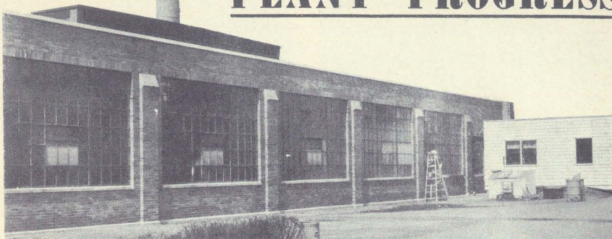
Plant's profile has been changed in recent weeks with the completion of a new 120' x 120' addition at the East End.
