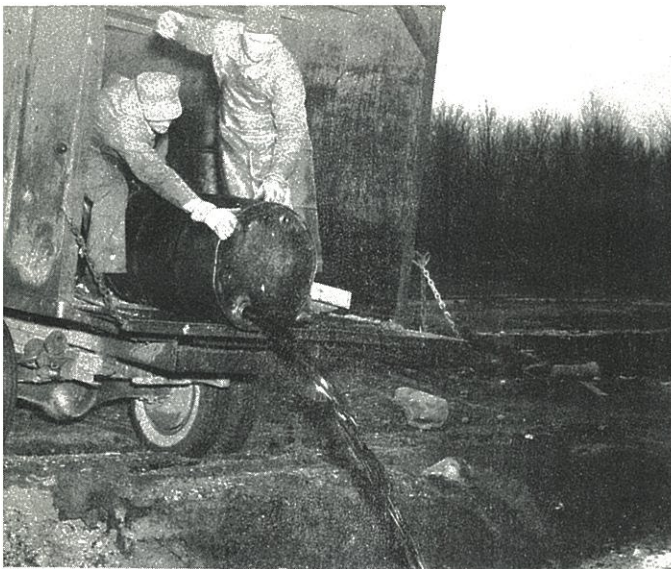
Ray Dean and Donald Teter are pictured here in the act of dumping a barrel of waste oil. Dumping is always rotated from used section of dump to unused so as to avoid possibility of highly inflammable thinners coming into contact with a fire which may still be smoldering from a previous trip.
