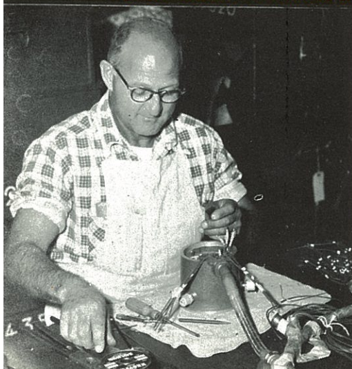
ROLAND HOOD of Dept. 47 completes wiring of harness to distributor.
