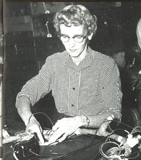
KAY GOSSOO attaches electrical connector to main wiring of harness.
