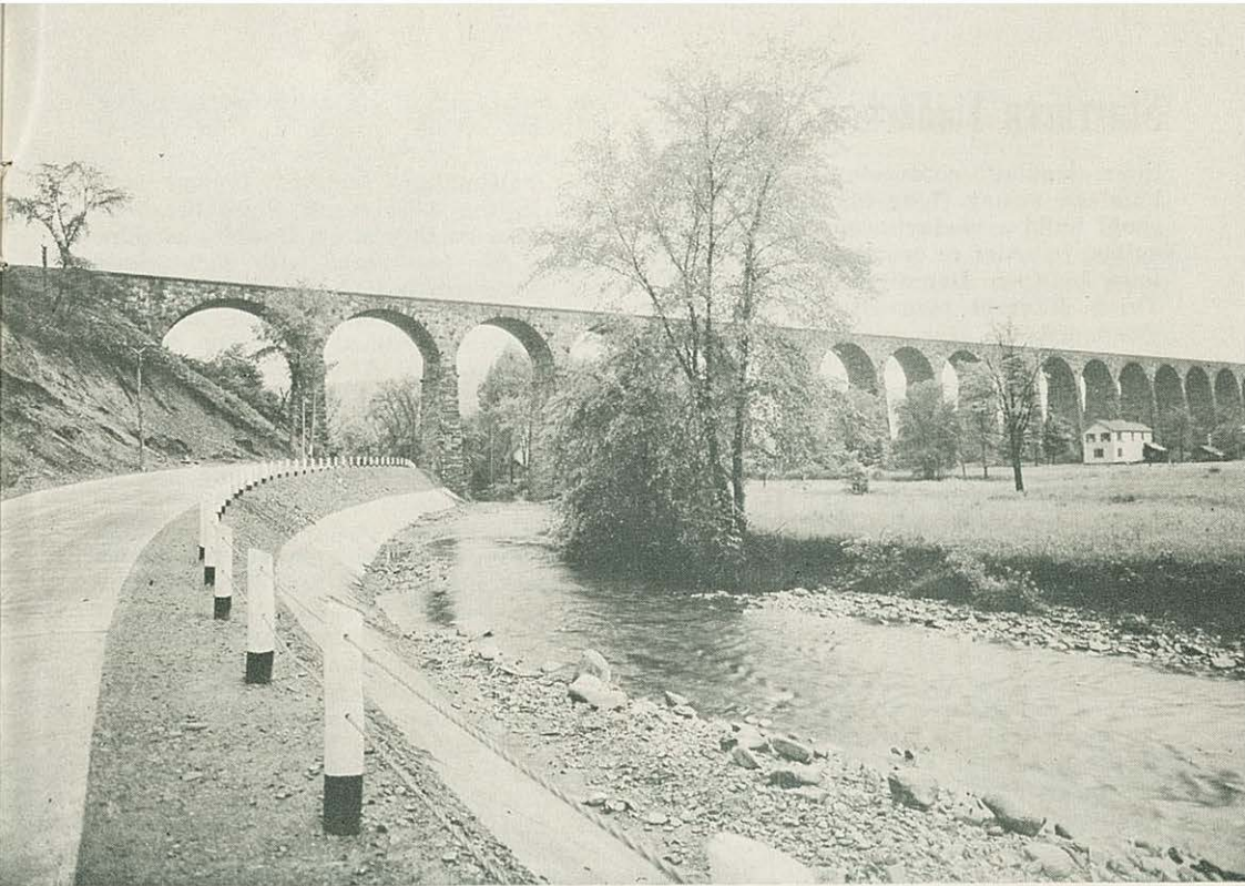
Listed as one of the wonders of the world is the Starrucca Viaduct, located at Lanesboro, Pa. Owned by the Erie Railroad, it was completed in 1848. It was built entirely of stone, with lime and sand mortar used as a binder, yet it supports today's heavy trains.
