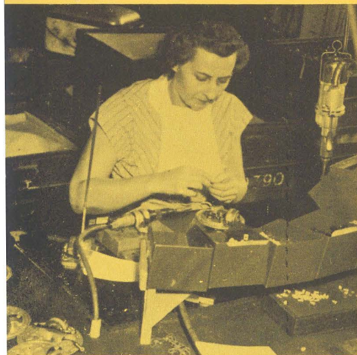
FLORENCE SABOR, Dept. 41, assembles the breaker and condenser to plate.
