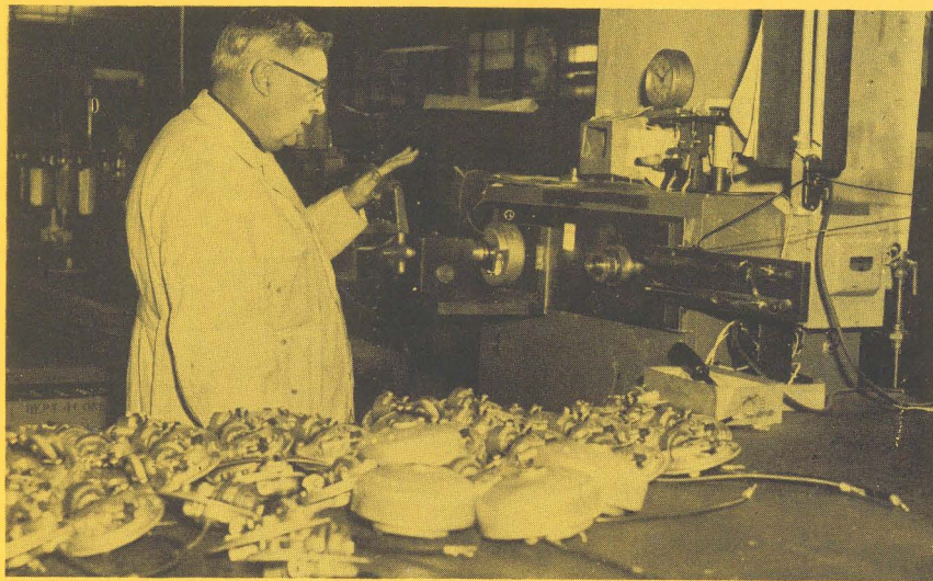
IN ONE of final steps, William Lord, Dept. 99, tests magnetos for spark.
