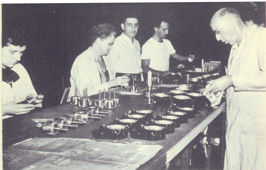
FINAL INSPECTION of rotors and tank magneto housings takes place in Dept. 40. Pictured—Lynn Duncan, Hazel McCoon, Bert Jeffers and Foreman Johnny Frank.
