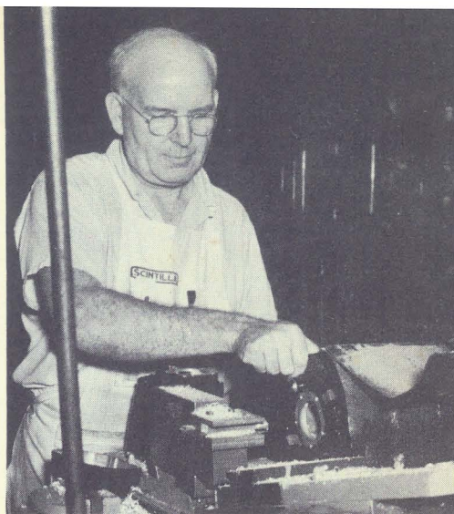
MILLARD PORTER loads housing cover into machine prior to boring.
