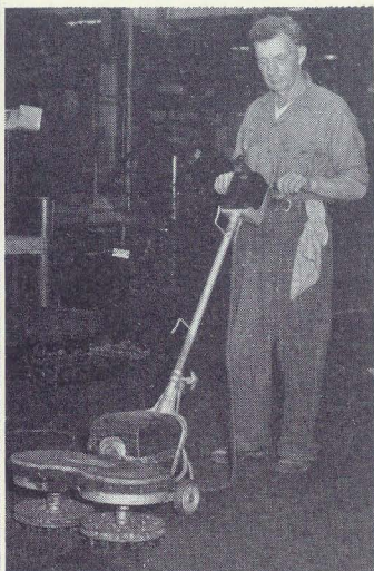
Below—William M. Merring runs Rover Dry Scrubber. Machine loosens chips, oil and dirt on floor.
