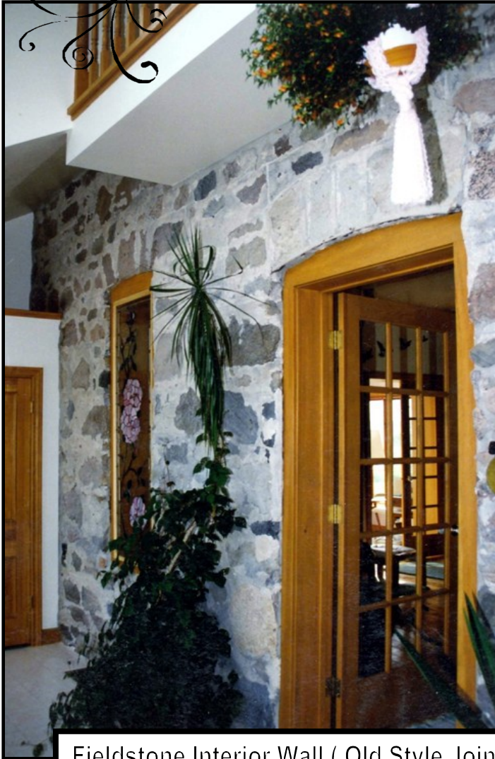
Fieldstone Interior Wall ( Old Style Joints )
