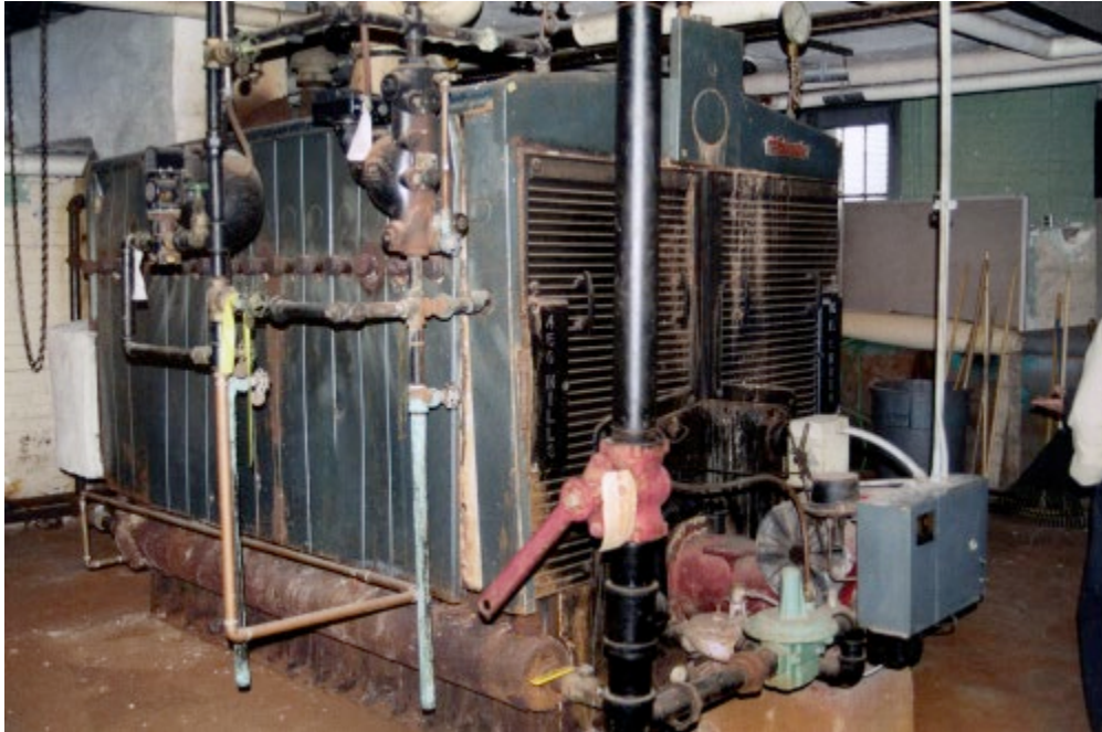
The Boiler Room in the basement of the Armory. A massive gas-fired Smith Boiler drove the steam heating system for the Armory plant. (photo: Arthur Motta, 2003)
